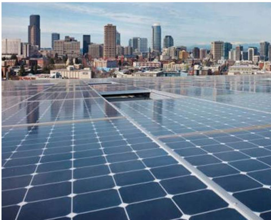
Figure 2. The Bullitt Center’s 242 KW PV (photovoltaic) array (Benjamin Benschneider).
